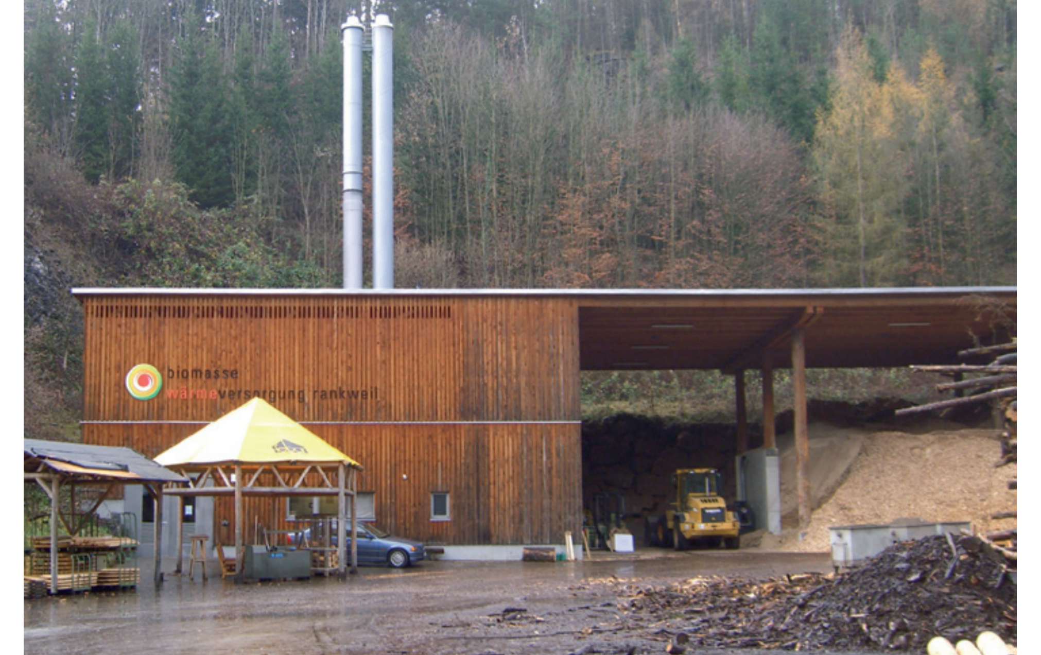
heating plant Rankweil, Austria
